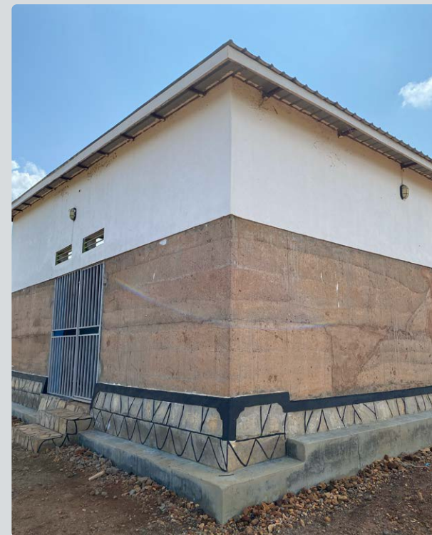
IMAGE 3. Pouring a soil mix into the rammed earth mould (12 Apr 2021, Pagirinya, Vuga William)
